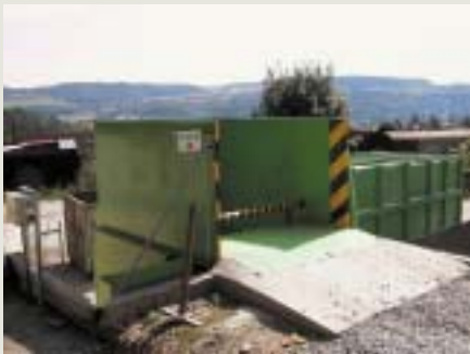
Drive-in ramp to SL1300 in a waste transfer station of household waste (TS Beroun)
