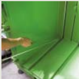
Preparation of strapping tape before pressing
